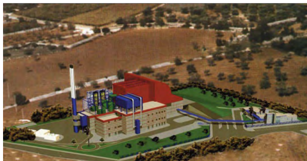
Lecce waste to energy plant
