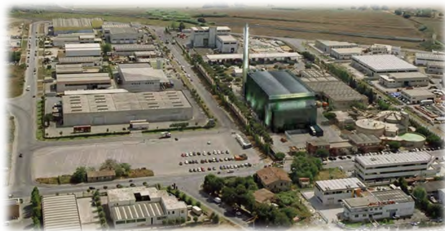
Leghorn waste to energy plant
