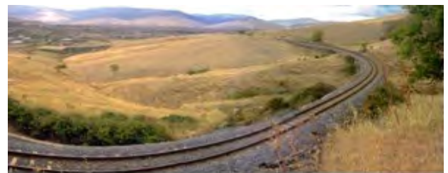
Viaduct "Brancatello" – Current
