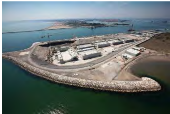
Chioggia inlet – Precast caissons yard
