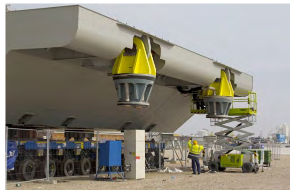
Steel mobile surge barriers
