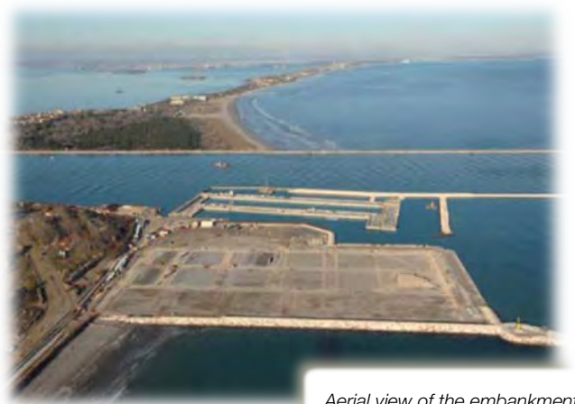
Aerial view of the embankment
