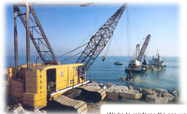
Works to reinforce the sea wall
