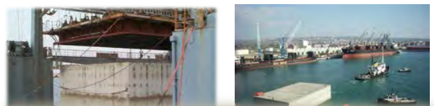
Typical phases of construction, launching and transportation of prefabricated elements
