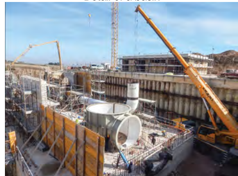
Detail of the main pipe construction
