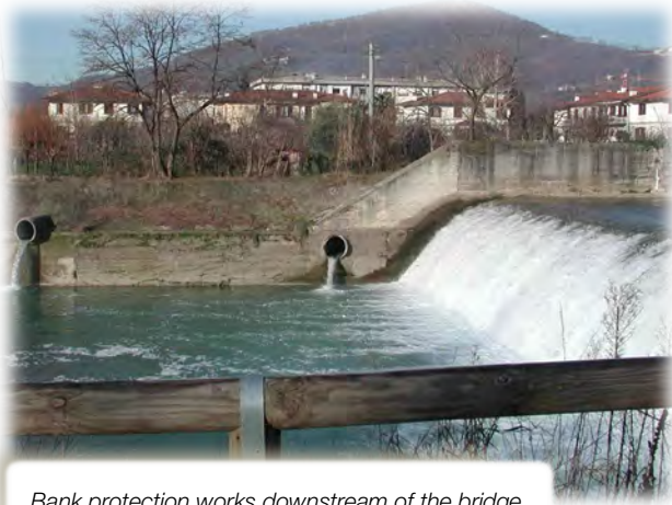
Bank protection works downstream of the bridge
