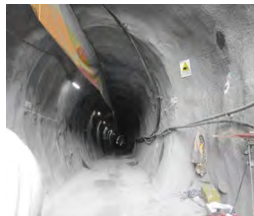
Bottom discharge tunnel of Miscuni Dam
