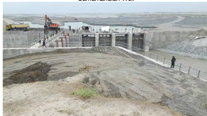
Yetim Tapa Channel Weir
