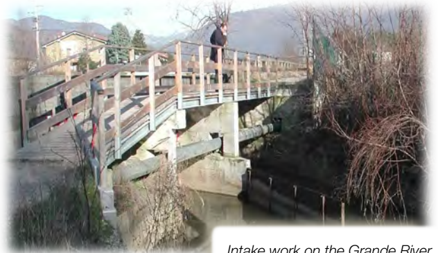
Intake work on the Grande River
