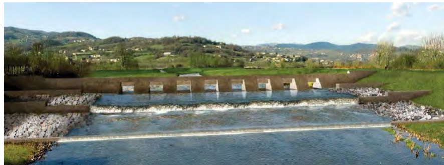
Eight gates connection structure
