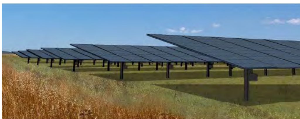
Rotello Solar power plants, Italy
