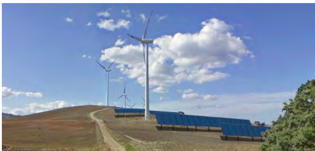
Rotello Solar power plants, Italy
