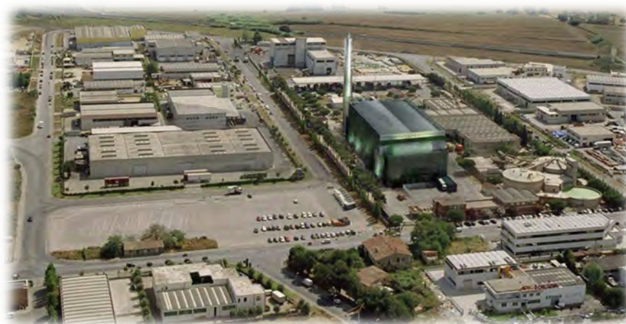
Leghorn waste to energy plant
