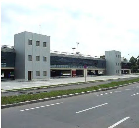
Multi-level car parking of Bucarest Otopeni Airport
