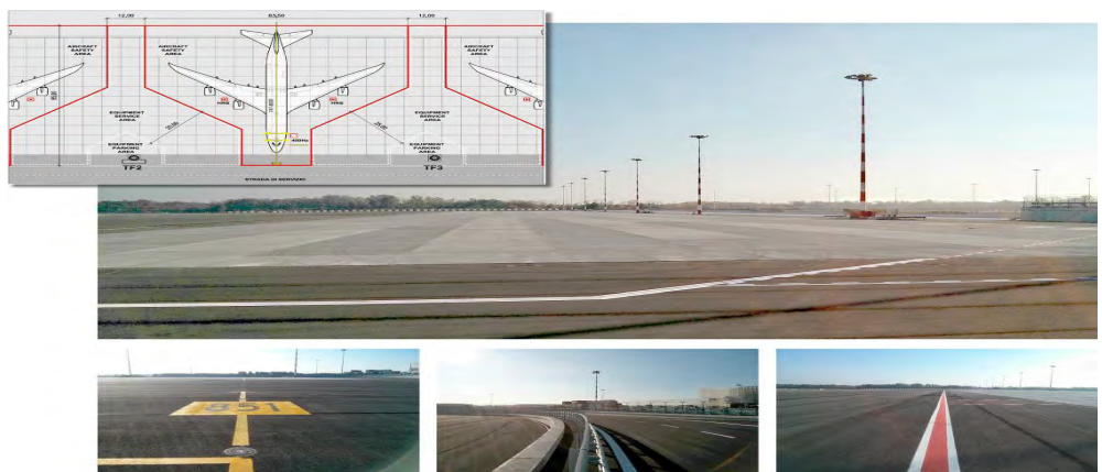
New cargo apron of Milan Malpensa Airport
